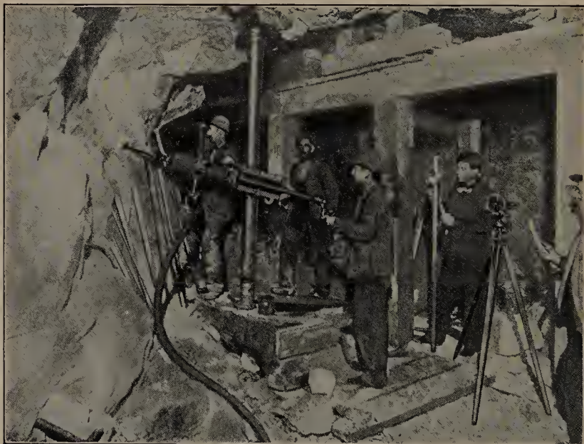
FIG. 193. Mining copper ore at Butte, Montana
